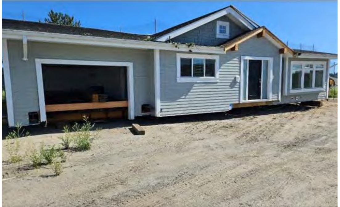
Temporary storage location for relocated houses at Lot 3 in Coquitlam Landfill
